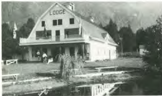
Blue Ridge Guest Ranch Lodge was later renovated to a barn pictured below.
