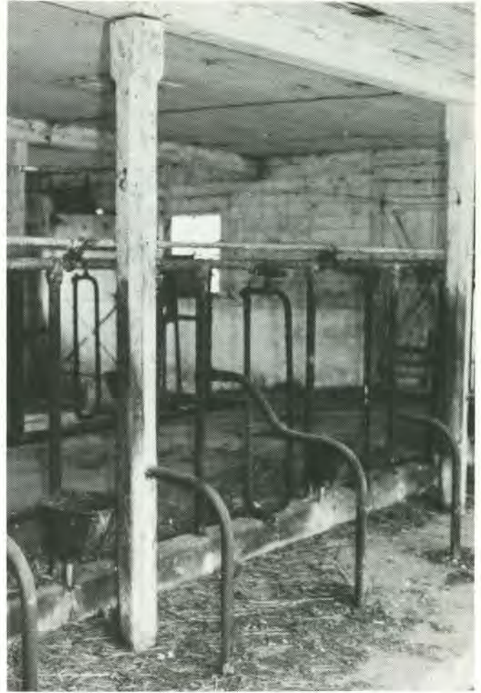
Interior of early stanchion barn, note posts and shaped concrete.
