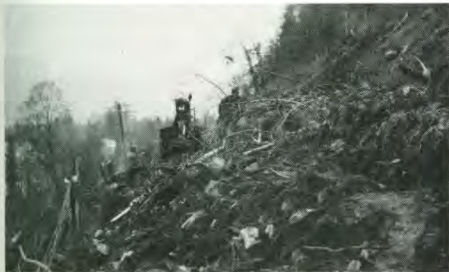
Slide clearing at Jones Hill.
