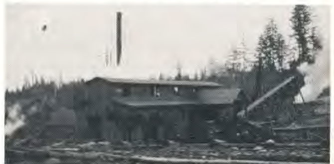
Below: The McNair Shingle Mill.
