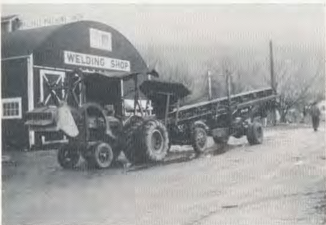
The first gravel loader designed and built by Rosedale Machine Shop.
