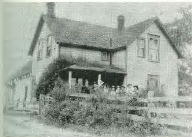
The Adachi Family Home at 10065 McGrath Road.
