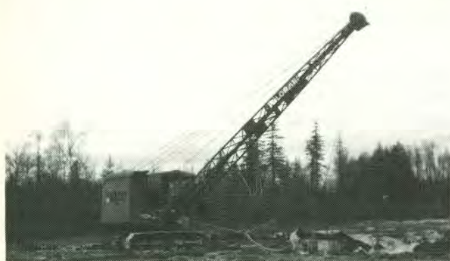
Dragline at Popkum Lake. (Cheam Marl Products).
