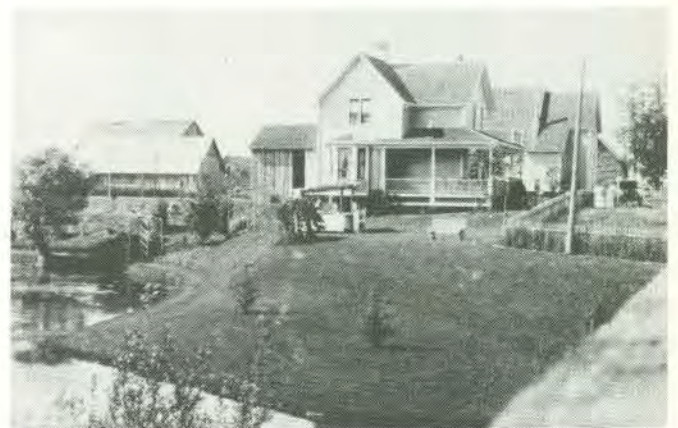
St. Peter's Rectory built by J. Martin, 1912.
