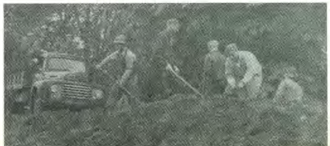
Below: Men working on the Rosedale dyke.
