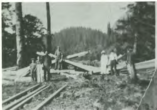
Start of construction of Herrling Island School.
