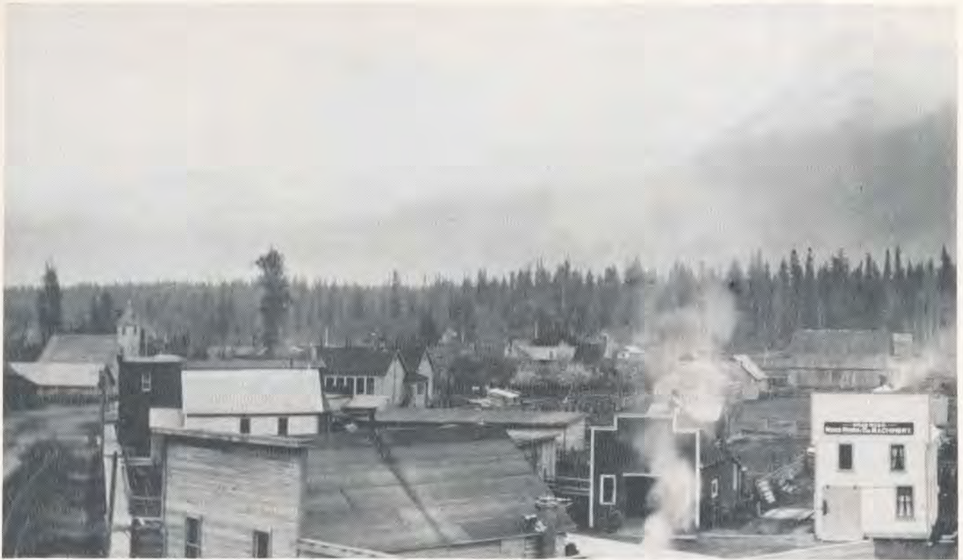
View of Rosedale about 1912 from roof of Somers Hotel.
