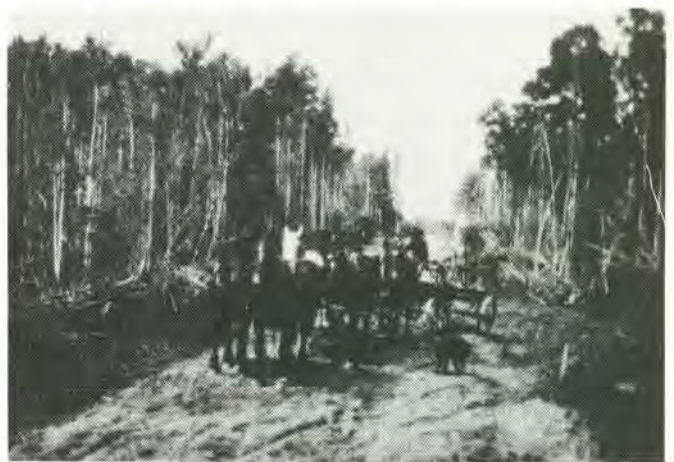
Early construction of Annis Road.
