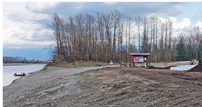
The Island 22 Boat Launch resloping project.
